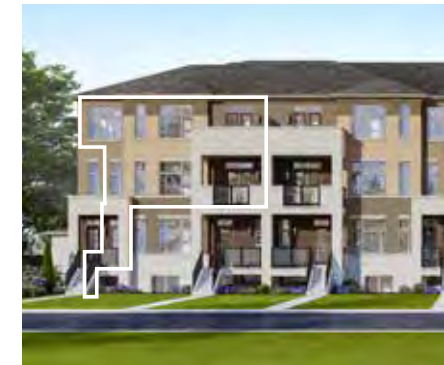
FRONT, Interior Unit
